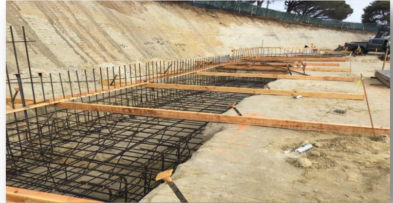
EWMS – Campus Re-Construction
