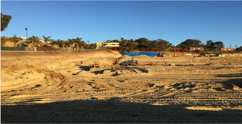
EWMS – Campus Re-Construction
